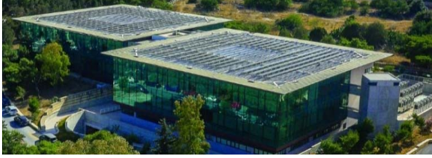
Fig. 2. Building testbed for the IoT big data capture and analysis system
